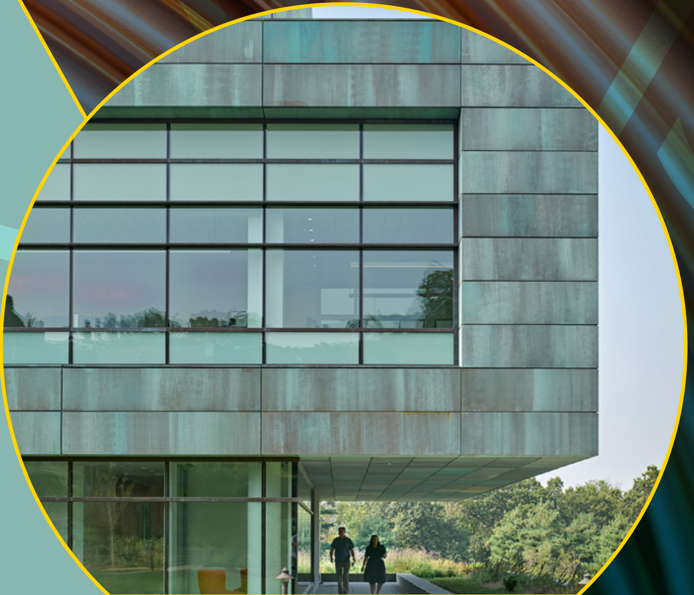
New England Biolabs Garden Site Facility Expansion Photo Credit: Robert Benson
