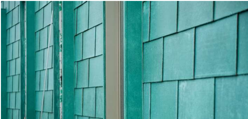
Detail of pre-patinated cladding panels. Image by Robert Umenhofer Photography.
