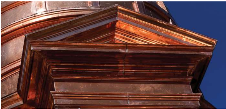
Detail of decorative roof element.
