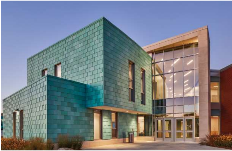
Day and evening views of plaza façade. Image by Robert Benson Photography.
