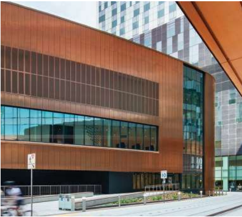
Amphitheatre façade and soffits opposite.
