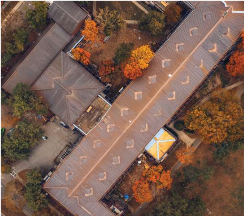
81,000 square foot copper roofs.
